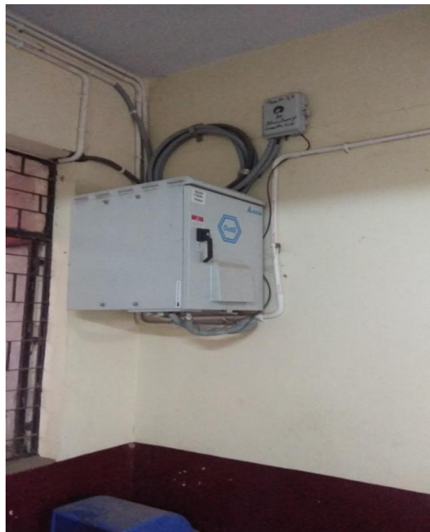
Switch used by Reliance Jio
