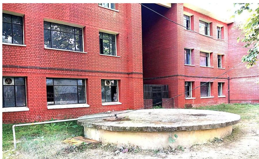
Figure 13 Underground roof top rain water harvesting tank
