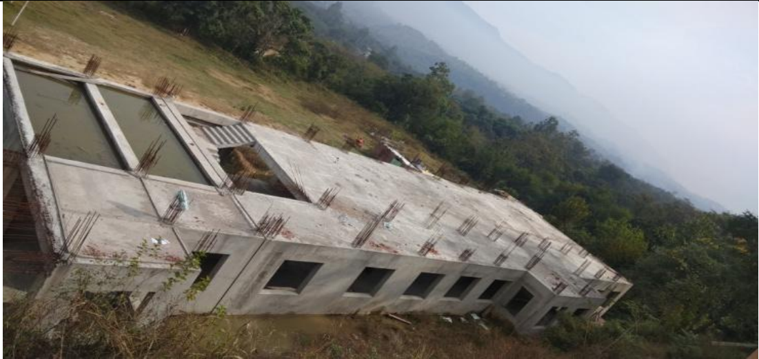
Construction of New Block
