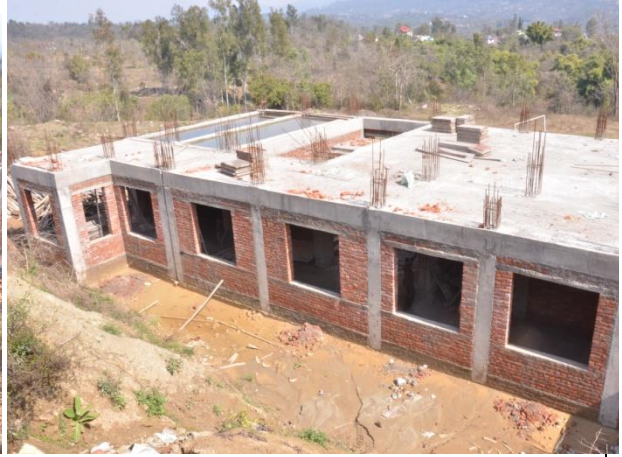
Construction of New Block
