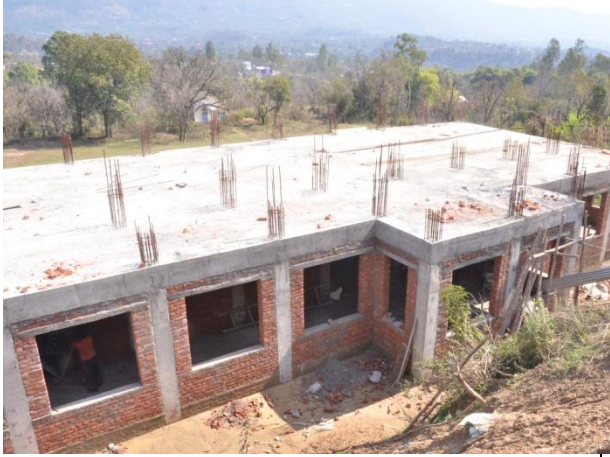
Construction of New Block
