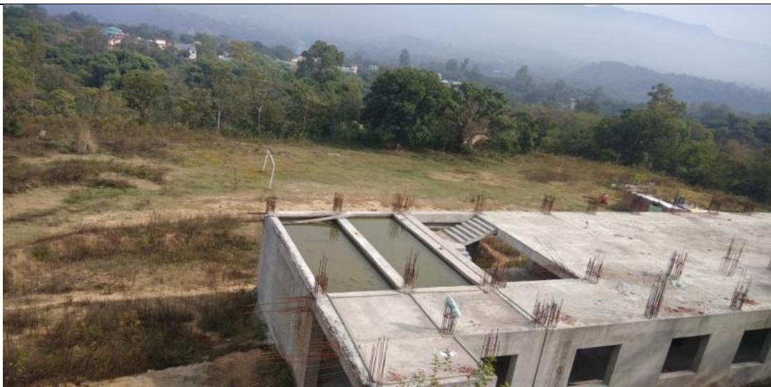
Construction of New Block
