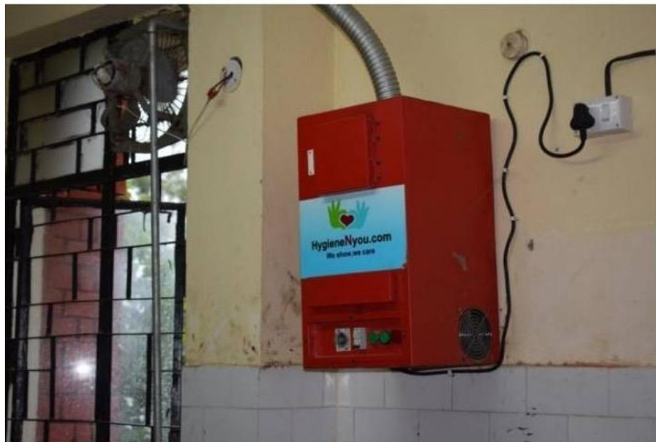
Fig. 6. Incinerator installed inside the girl's washroom.
