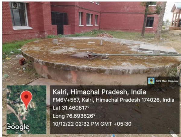
Fig: 9. Underground roof top rain water harvesting tank.
