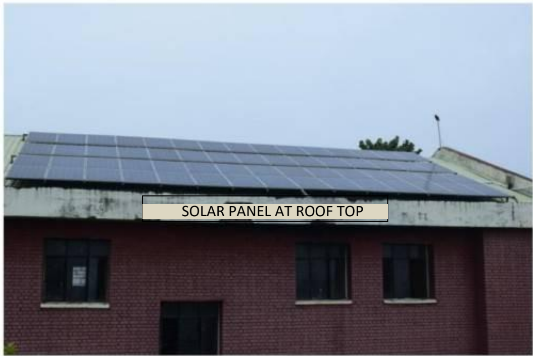
Fig: 10. Solar panels installed on the roof of college building.
