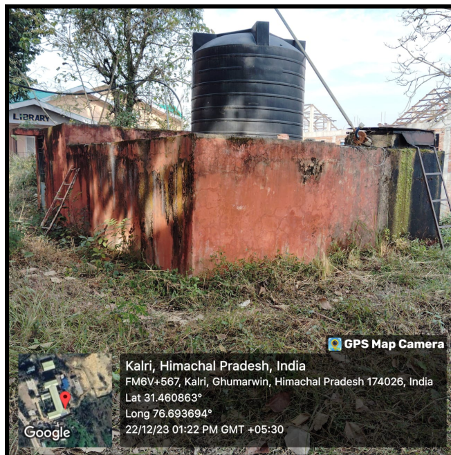
Water Storage Tank
