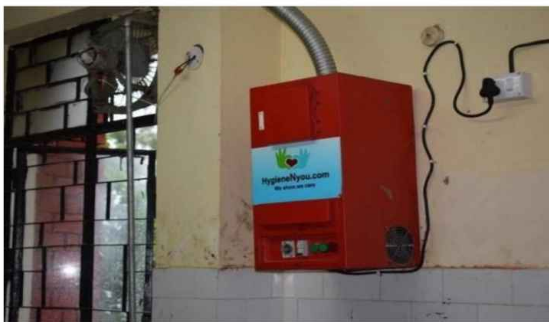
Incinerator installed inside the girl's washroom
