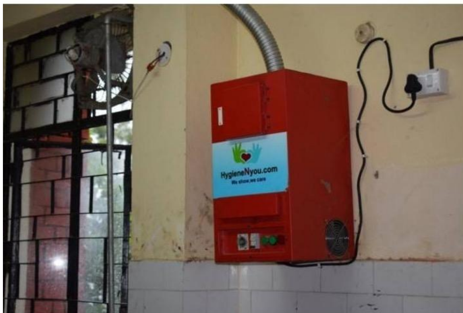
Incinerator installed inside the girl's washroom.
